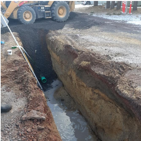
Figure 1: Image of a mainline trenchwork along the south Main st line.
