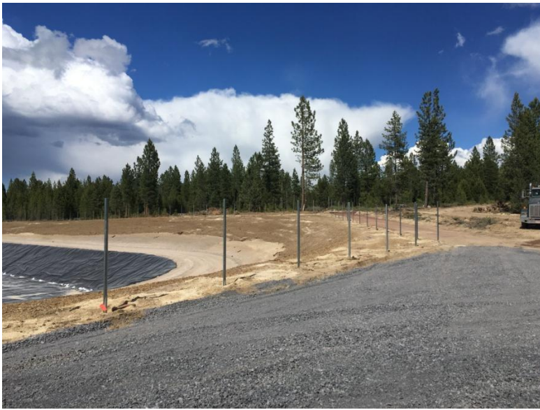
Figure 9: Looking north at the newly gravelled entrance road and fence poles running the perimeter of the facility.
