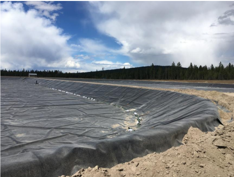
Figure 4: Looking northeast at both lagoons. Note that they are both completely lined.
