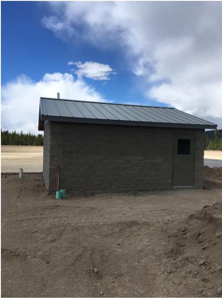
Figure 6: Looking north at the completed roof on the chlorinator building.
