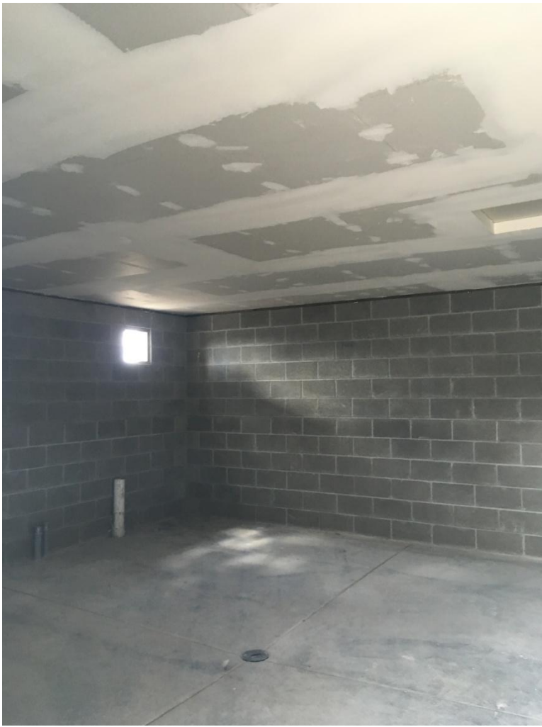
Figure 7: Looking inside the chlorinator building at the completed ceiling.
