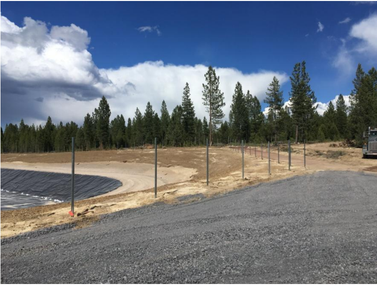
Figure 9: Looking north at the newly gravelled entrance road and fence poles running the perimeter of the facility.
