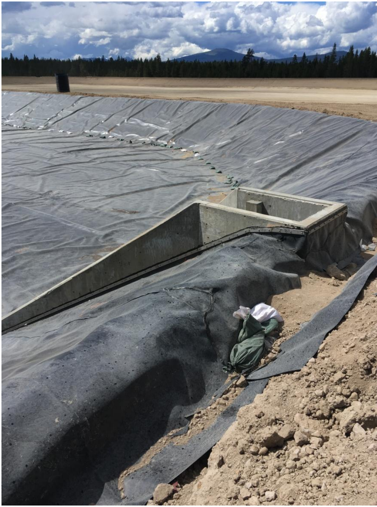
Figure 5: Looking northwest at the western lagoon that is lined. Note that the liner is bolted to the crossflow structure walls to ensure a complete seal.
