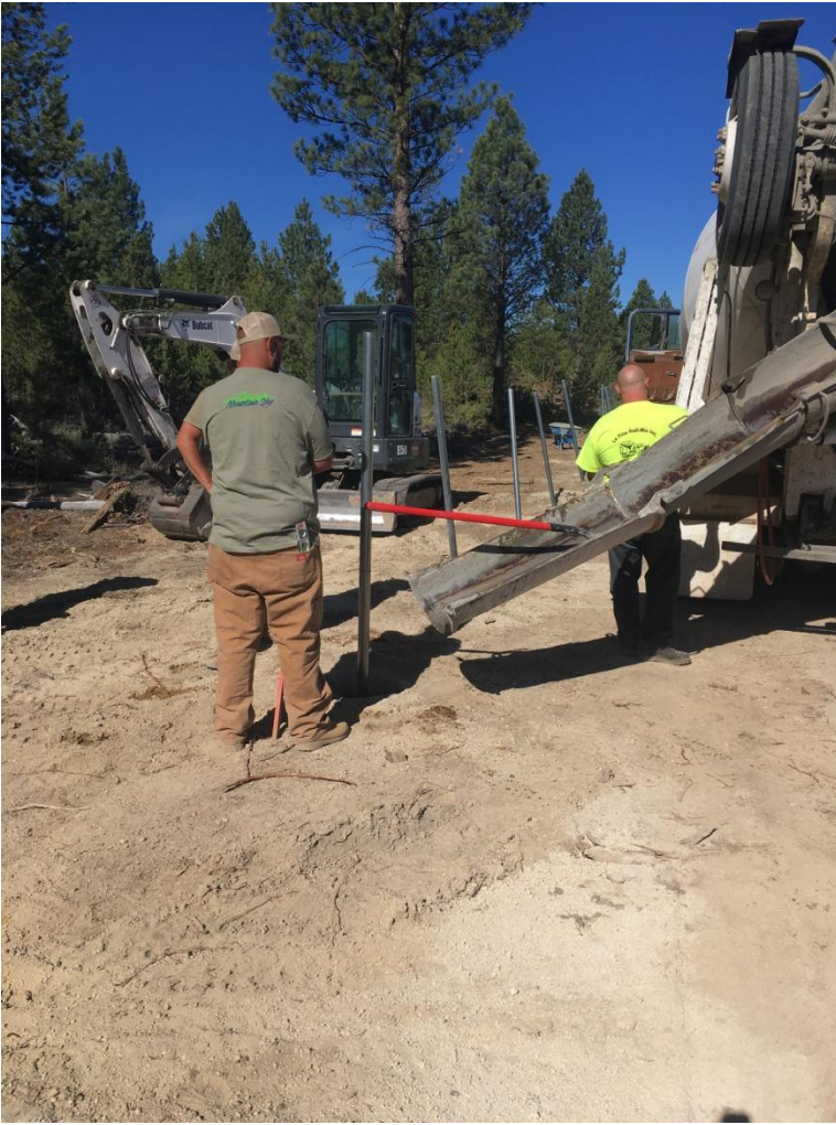
Figure 6: Image of fence posting being cemented into place.
