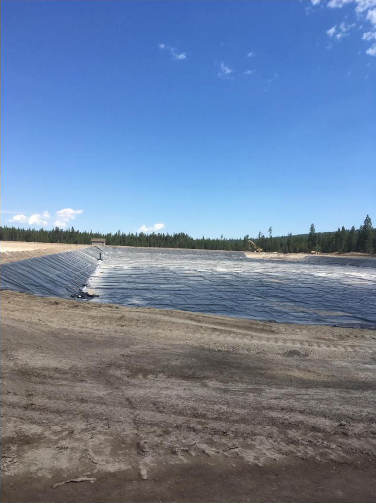
Figure 5: Looking north at the lined eastern lagoon.
