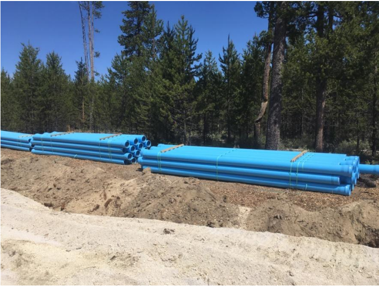
Figure 4: Water line pipes are on hand and awaiting installation.
