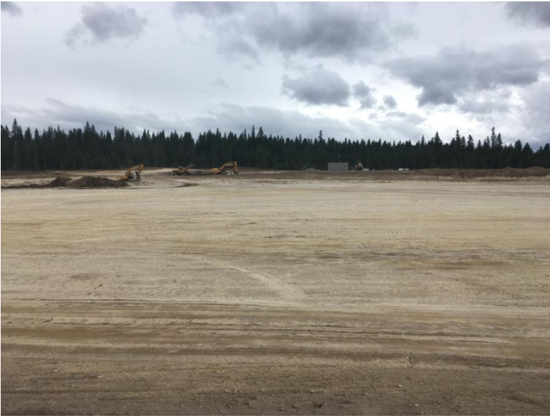
Figure 2: Looking east at the graded bottom of the storage pond.
