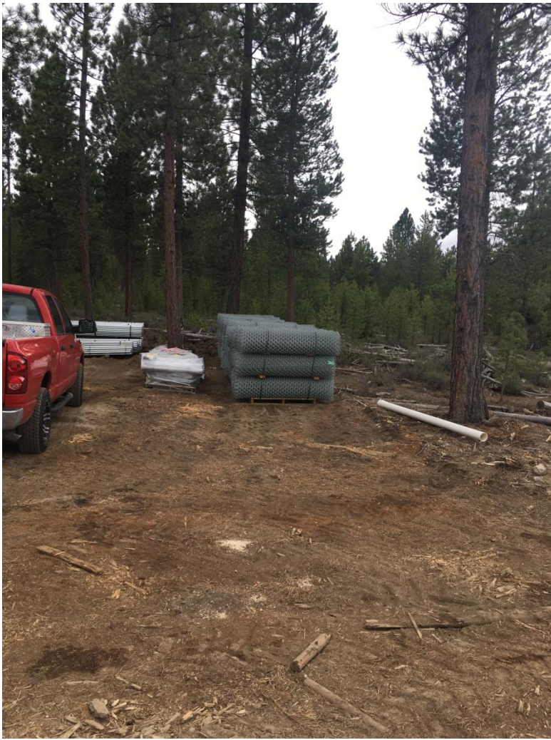
Figure 4: Fencing material on site and awaiting scheduling.
