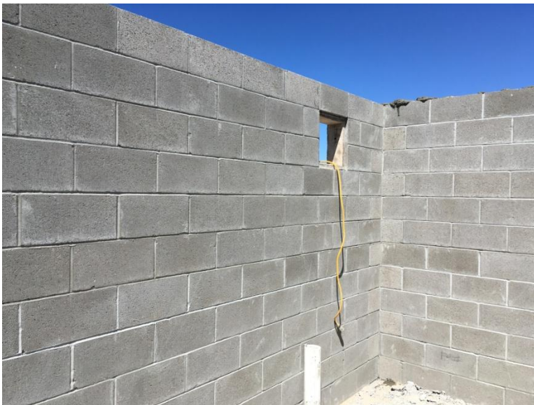
Figure 1: Looking at the top of the walls within the chlorination building. Note the threads protruding at the top of the wall, this is where the roof will attached to the building.
