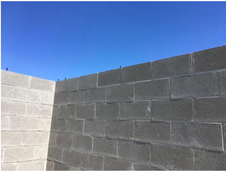
Figure 1: Looking at the top of the walls within the chlorination building. Note the threads protruding at the top of the wall, this is where the roof will attached to the building.
