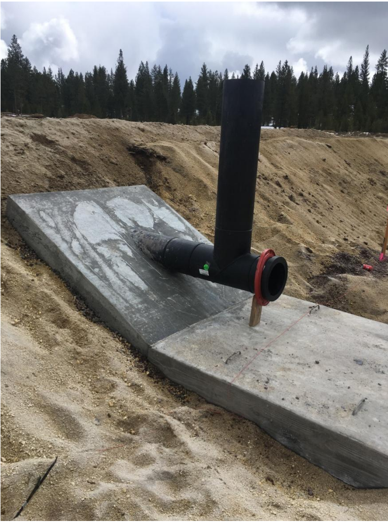
Figure 6: Communication crossflow structure rat wall (western).
