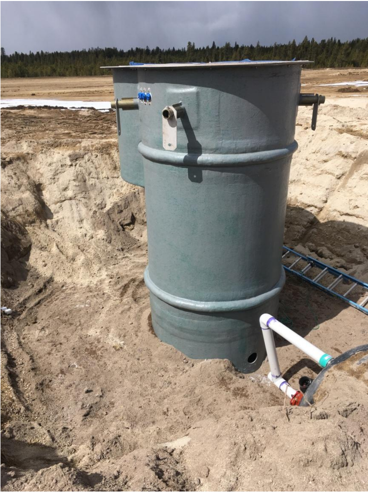
Figure 4: Looking northwest at the installed lift station.
