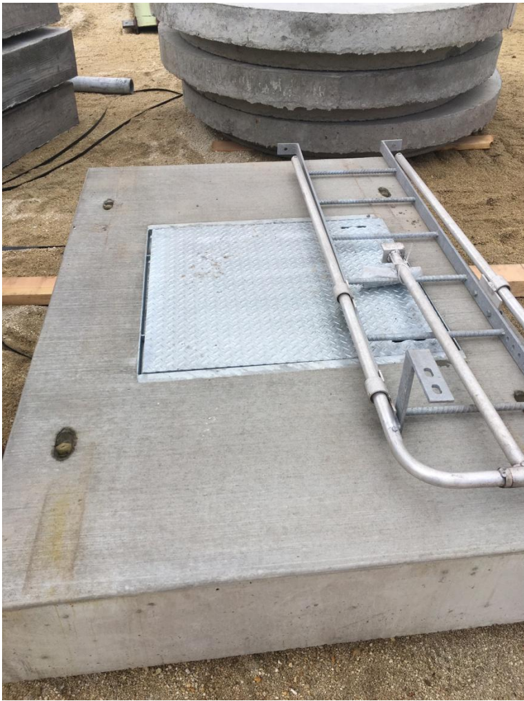
Figure 7: Materials on site.
