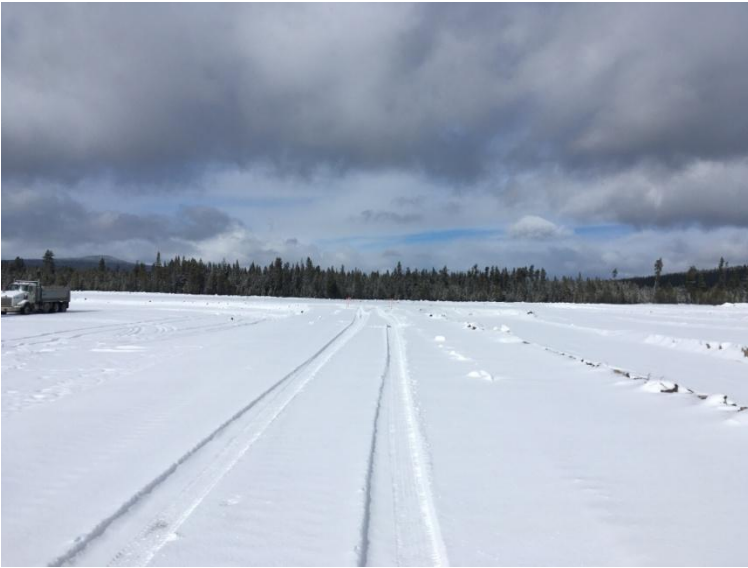
Figure 5: Looking north, far in the background one can see five stakes delineating the location of the 3 risers, and pipe centers between the risers for the chlorinator.
