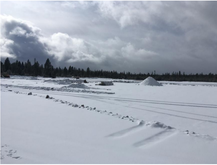
Figure 3: Looking northwest at the western lagoon. Note the pipe laid out in the center of the picture.
