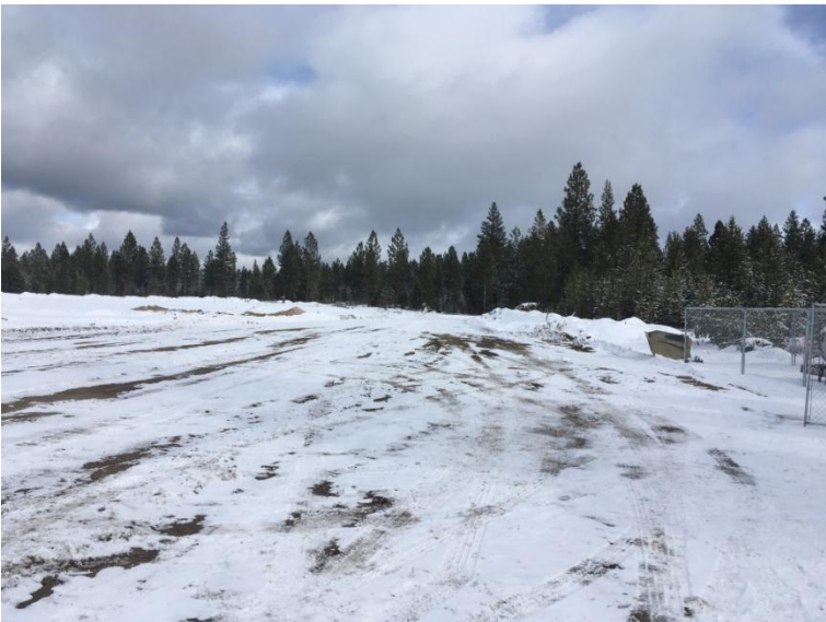
Figure 2: Looking east at the edge of the eastern lagoon. Access road into the job site is in the background.
