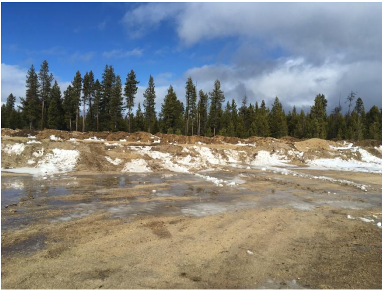
Figure 4: Looking northwest at the storage pond. Note the staging of build up materials. The “darker” piles consist of a lithology more amenable to supporting the berms.
