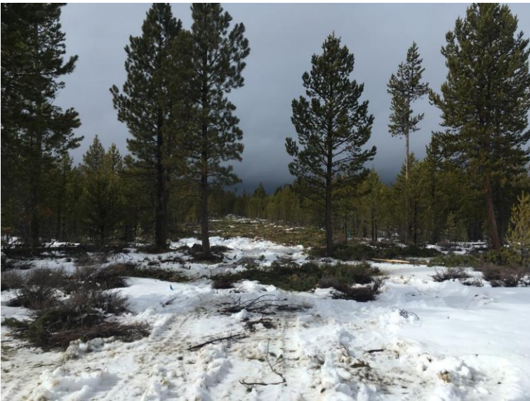
Figure 5: Looking west at the grubbed irrigation main line.
