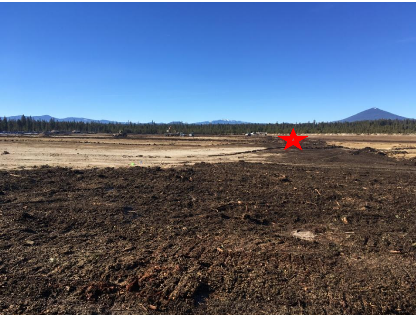
Figure 2: Looking West at the conduit between the lagoons and the storage pond. The star marks the approximate future location of the Chlorination Building.
