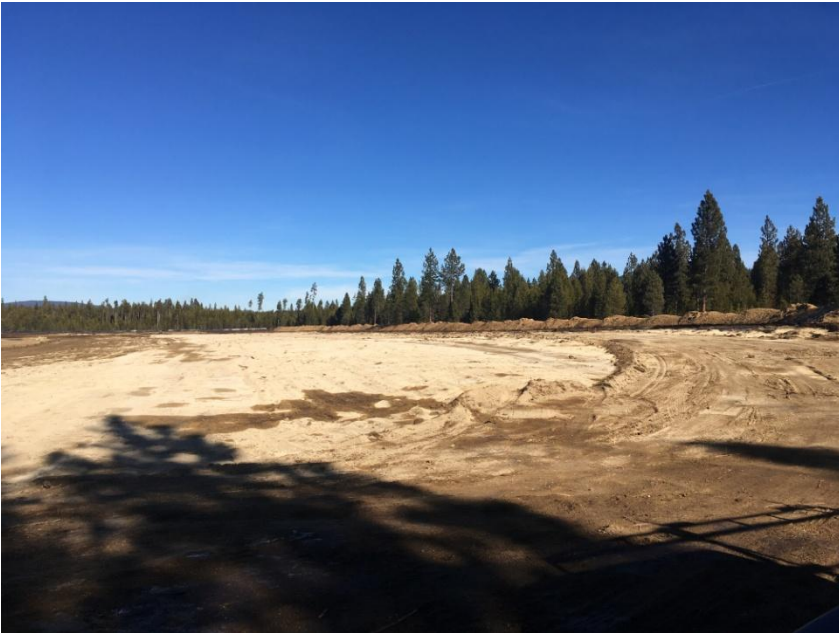
Figure 1: Looking North at the eastern lagoon. Note the start of the berm build up on its eastern boundary.
