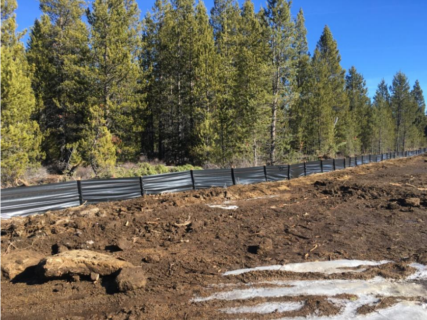
Figure 4: Looking northwest, at the western boundary silt fence.
