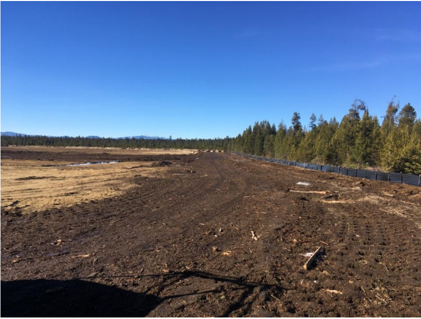
Figure 3: Looking West at the northern boundary silt fence.
